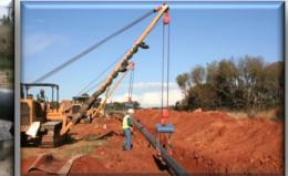
PL4 (Anglo Coal Section) Pipe stringing and bending completed at the Anglo Coal Section. **3.8km** has been welded, coated and ready for lowering-in.
