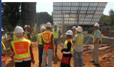
Solar panels, keeping it green all the way.
