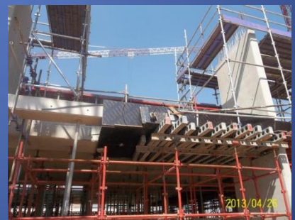
Staging and formwork.
