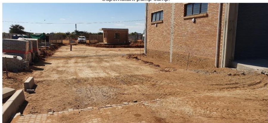
Layer works around machine room.
