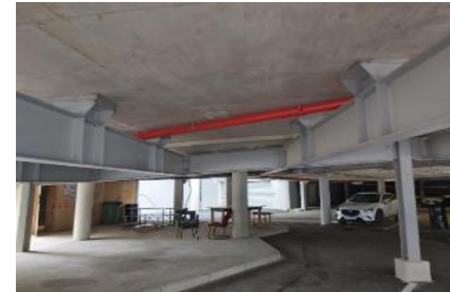
Steal beams used to strengthen ramp designed with insufficient load-carrying capacity
