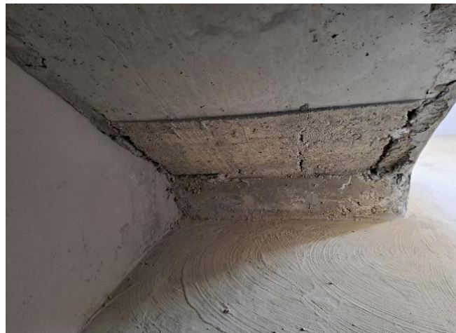
Figure 1 & 2: : Cracks on honeycombing underneath the staircase
