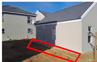
Vlakkeland (Paarl) housing project (WC Department of Human Settlements): Houses founded at incorrect level – vulnerable to stormwater flooding
