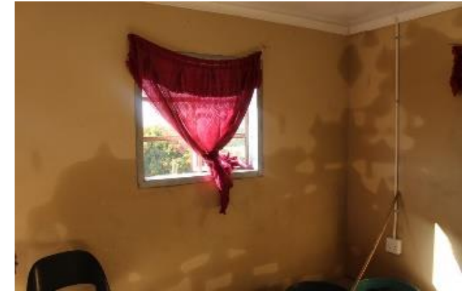
Figure 3: Water penetration on internal walls
