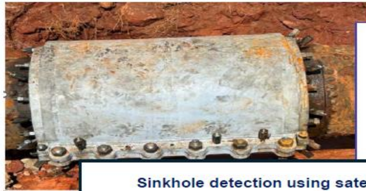
Non-interruptive leak repair
